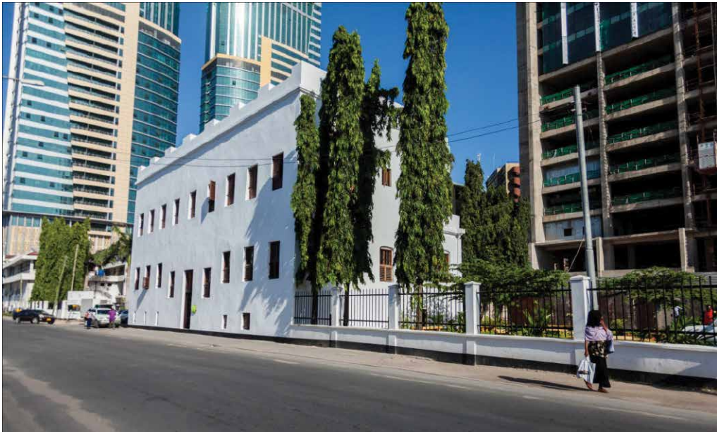
The Old Boma after refurbishment
